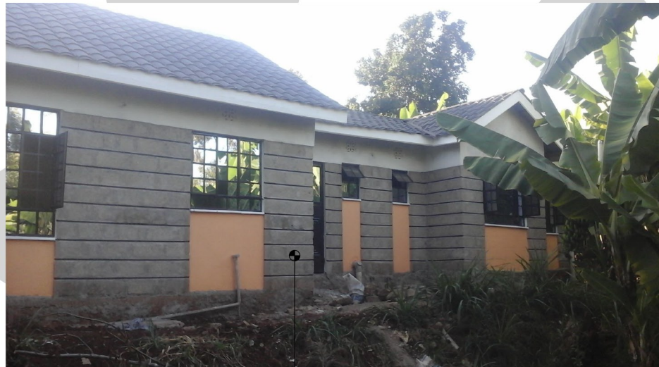
SHOWING BACKSIDE OF CONSTRUCTED HOUSE
